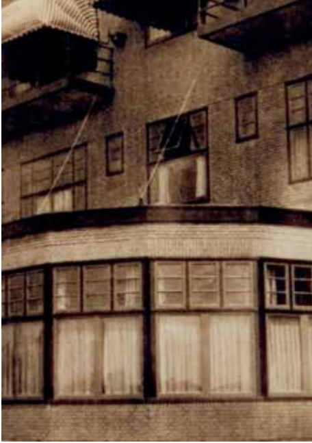
Figure 3.7: The back side, just after completion in 1929, showing the annex and the two cables by which the roof could be elevated during Sukkot.
