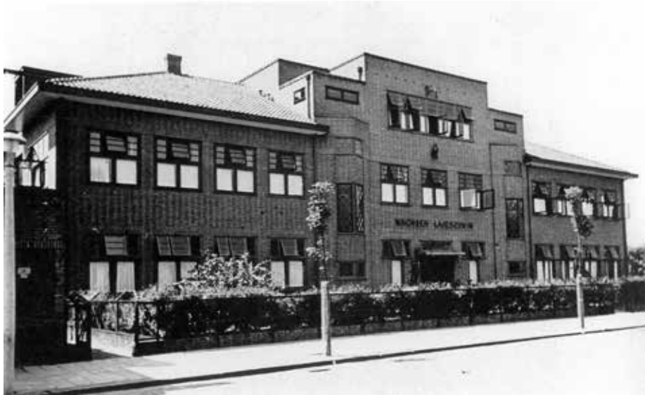
Figure 3.2: The front side of the new building, probably 1930-1931 (see text and design drawings).
